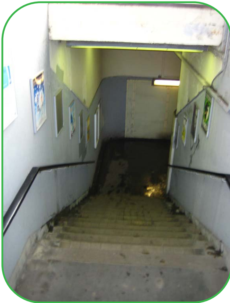
Photograph 1 – South Ruislip Underpass
