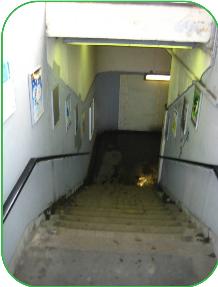
Photograph 1 – South Ruislip Underpass
