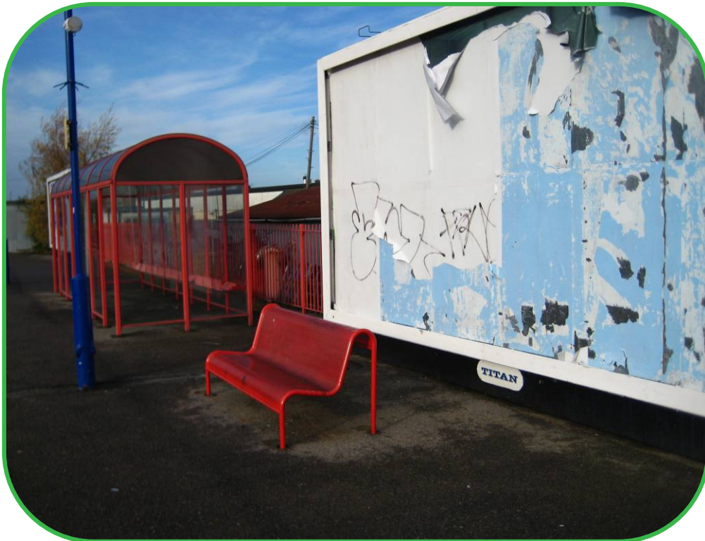
Photograph 3 – South Ruislip Waiting Facilities
